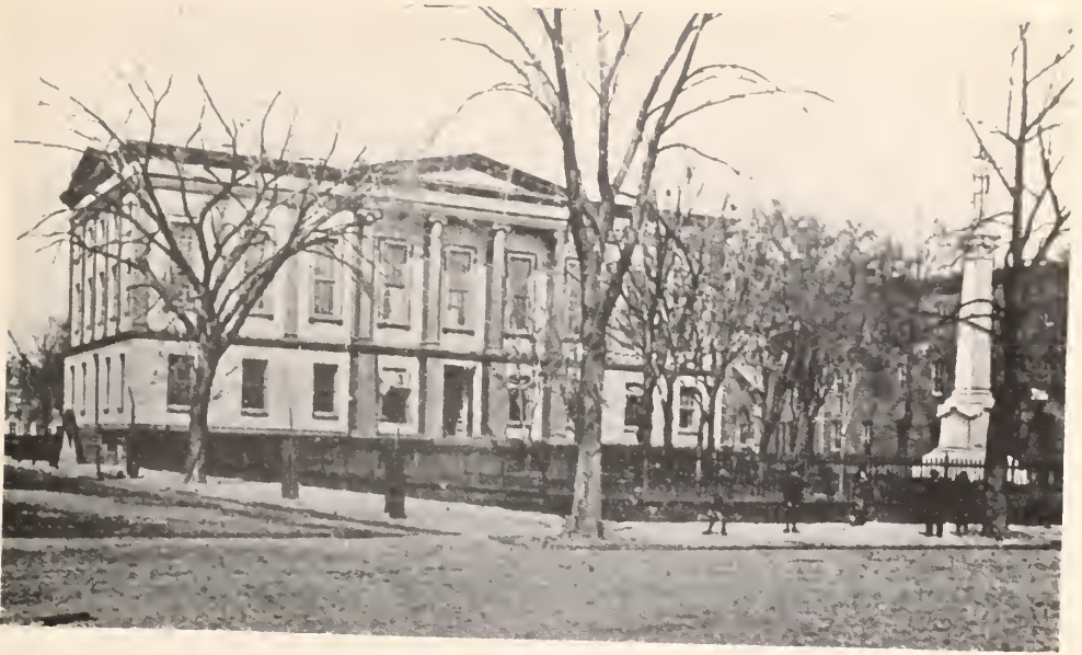
SECOND COURT HOUSE, CAMDEN
